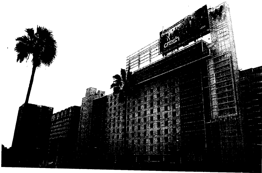
A new mixed-use transit-oriented development has been built on the Hollywood and Vine Metro Red Line Station. Photo by Alek Friedman
